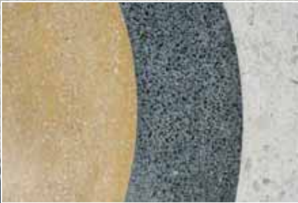
The upper part was closed with yellow concrete bordered by a blue-grey concrete ring.
