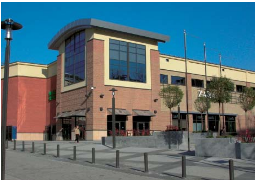
– the hollow blocks and bricks in the facade are made of AALBORG WHITE® cement.
