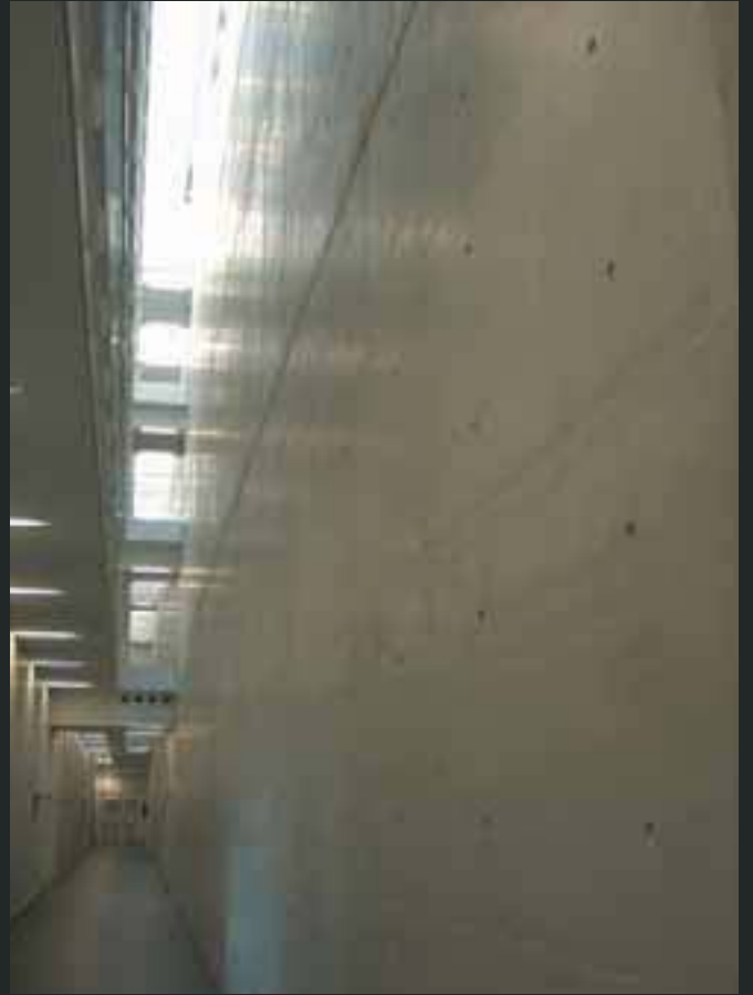
The building's solid vertical white concrete spinal column, which spans all the building's 14 storeys and, both practically and aesthetically, unites the building's main functions.
