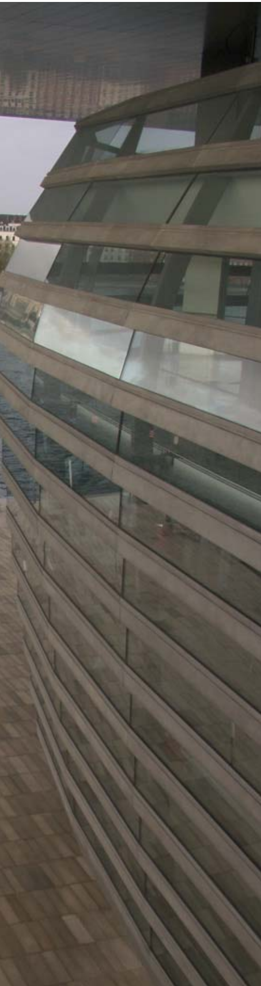
The outer surfaces of this gigantic core were constructed as a careful combination of concrete poured in situ and modular concrete.
