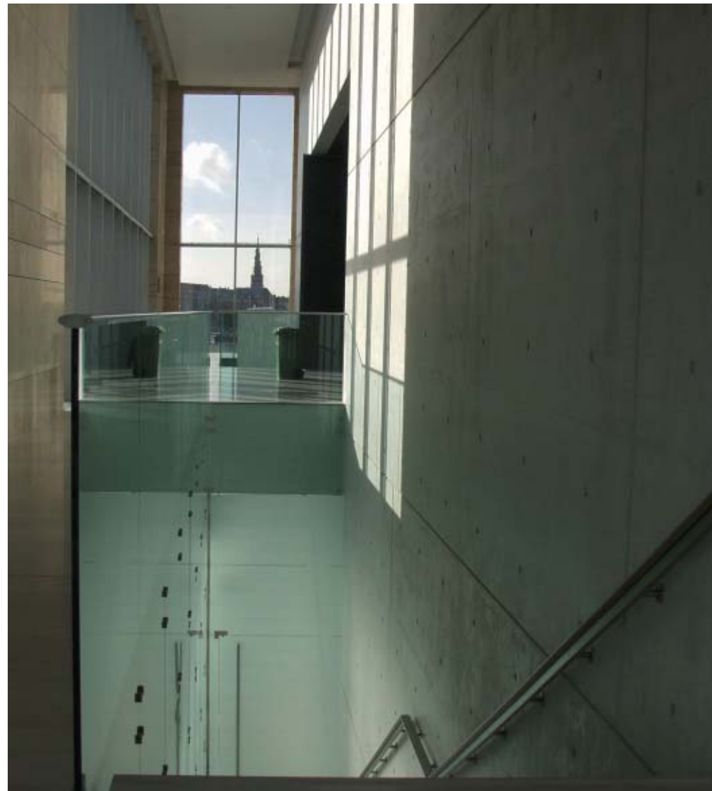
The outer surfaces of this gigantic core were constructed as a careful combination of concrete poured in situ and modular concrete.
