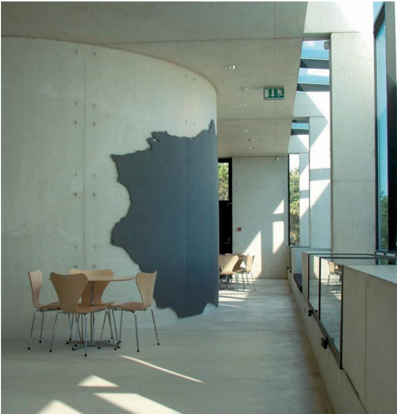
The colours and materials used in the interior highlight the fine white in-situ concrete in intelligent interplay with light-coloured birch panelling.
