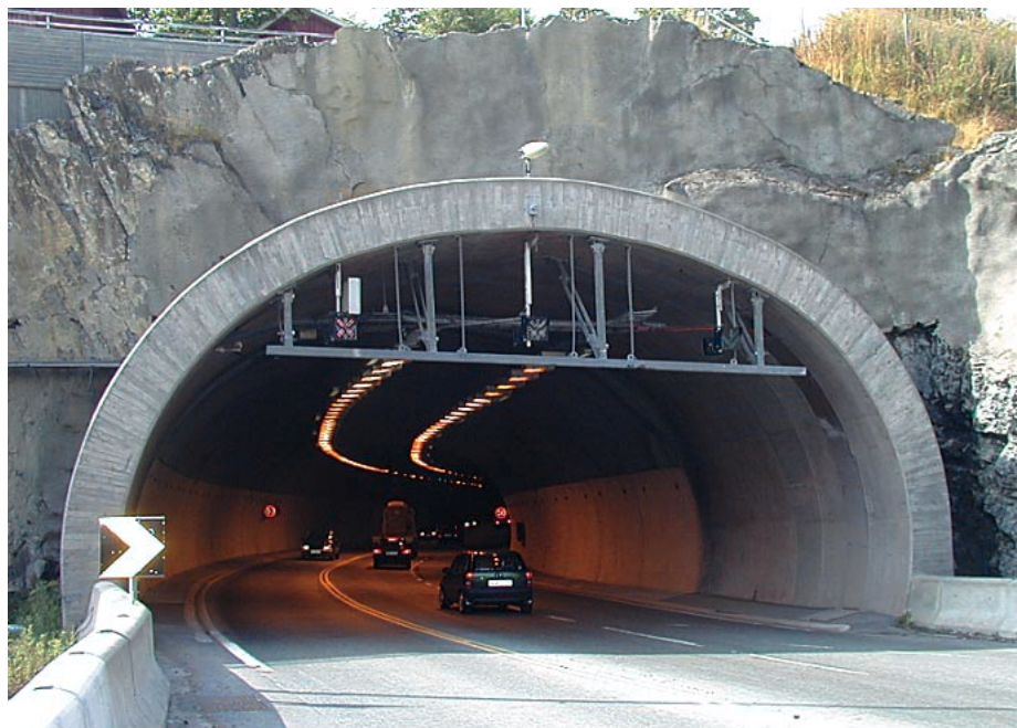
Greater reflection in the tunnel improves road safety.
