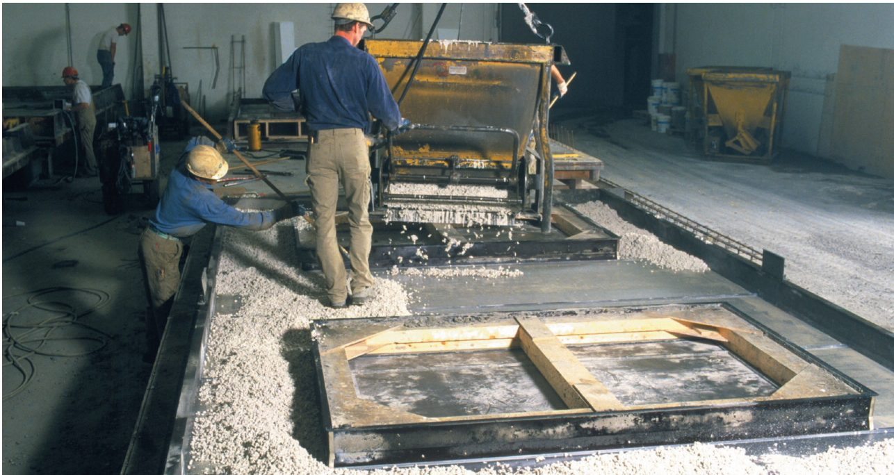
Vibrating table for concrete elements for facings.
