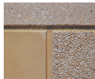
Polished, acid-etched and exposed surface with Glen Sanda 4/8 (Scottish aggregate).
